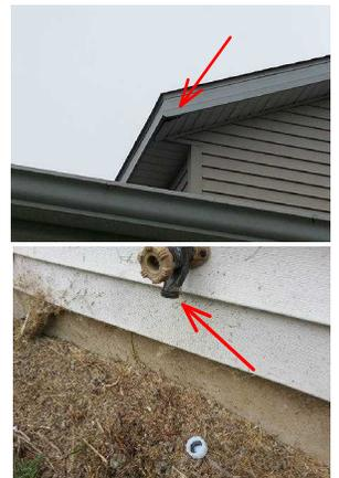
23. Hose Bibs: I observed two hose faucets. The rear hose faucet dripped constantly, even when turned off. It had a cap installed on it to prevent dripping. I removed the cap to prevent possible further damage to the faucet from upcoming freezing weather. Have repaired by licensed plumber.
