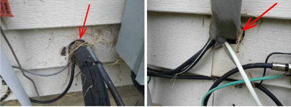
26. **Exterior Vents** The round vent covers used on the lower rear walls were not well sealed and did not have screening installed. Better sealing vent covers should be installed in these locations, to keep out water and possibly pests. (replace 3 vent covers)
