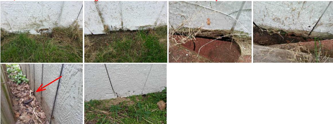
33. Back yard Outbuilding Doors: **The wood doors were decayed at the bottom, and nails stuck out where boards have fallen off. The pointed nail heads could be a hazard.**
