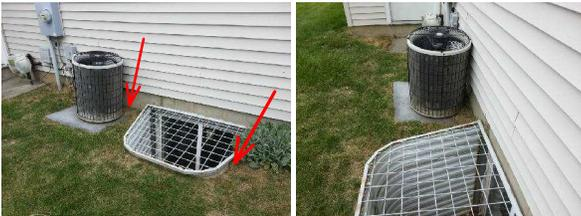
31. Window Wells: **Remove excess soil from the window well (the surface of the soil or stone should be well BELOW the window, to help prevent water entry).**
