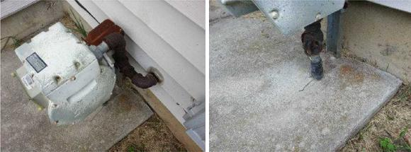
25. **Exterior Sealing** Caulk needed, where air conditioning lines entered the house. Caulk needed, where electric service enters house, to exclude the elements.
