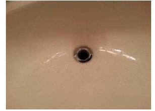
13. 2nd floor master Bathroom Spa Tub/Surround: **Whirlpool was filled and operated. I could not find any indication that the whirlpool tub was properly GFCI protected. Proper protection should be verified by a licensed electrician.**
